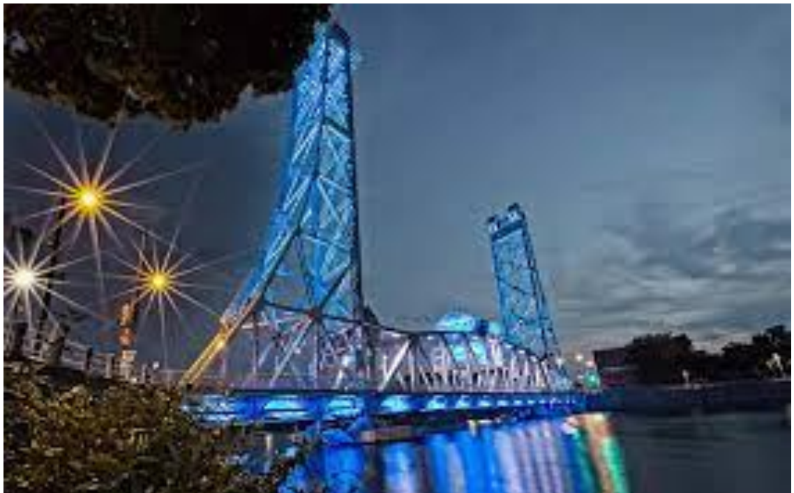
The East Main Street bridge – a local landmark.
